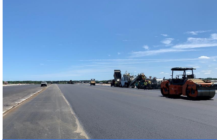
Asphalt Leveling & Paving
