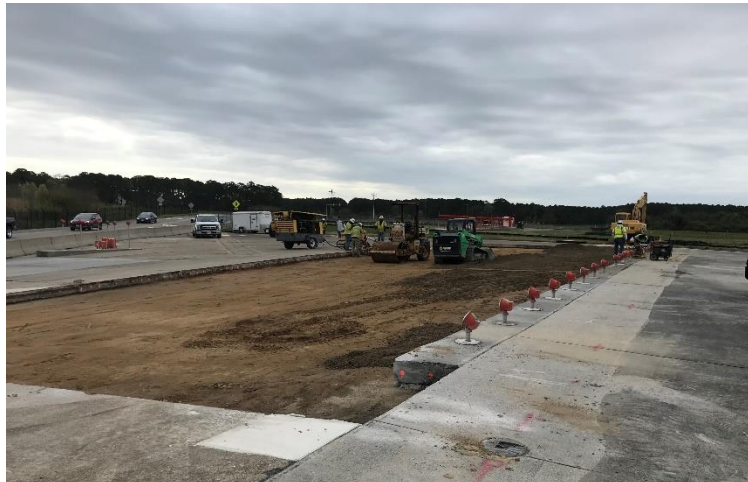
Concrete Repair & Joint Sealing
