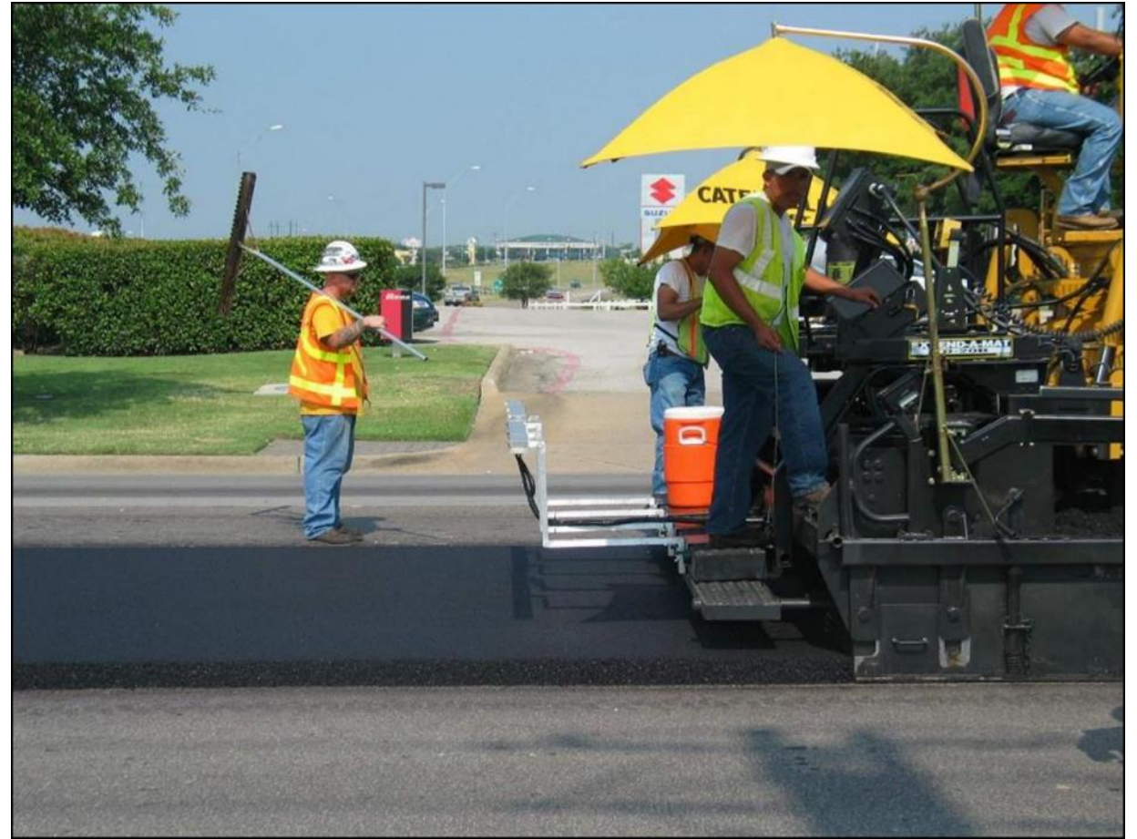
CORRECT SQUARE JOINT — END GATE DOWN
