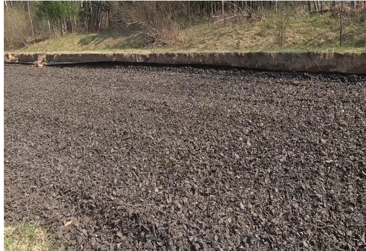
6 inches of tire-derived aggregate in Clare County construction, MI
